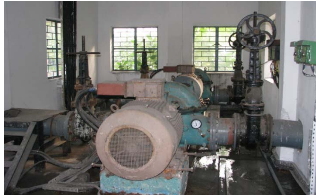
RECIRCULATION PUMPS for Bottom Ash Handling System
