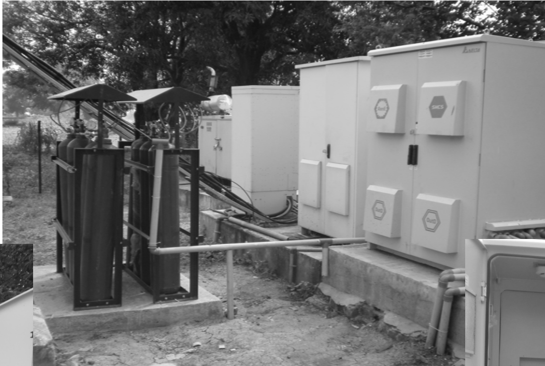
Site Monitoring & Control System
