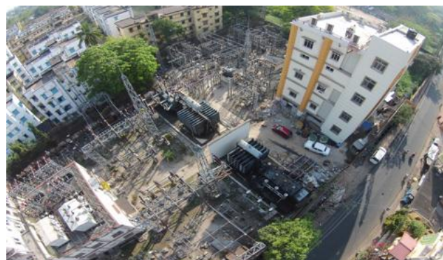
Conversion of Outdoor EHV SS to Indoor GIS SS
