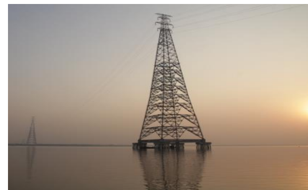
India's tallest Power Transmission Towers across Hoogly River (236m tall)
