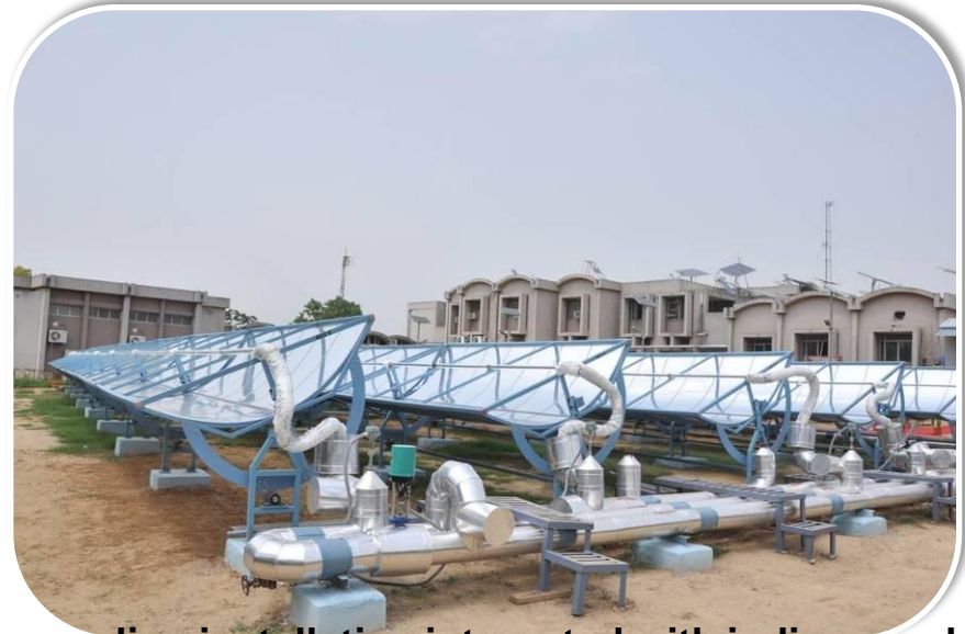
Solar Cooling at SEC, Gurgaon- FOAK triple effect solar cooling installation integrated with indigenously developed parabolic troughs by Thermax delivering 100 KW cooling
