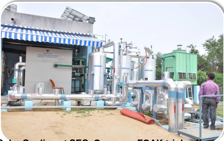
Solar Cooling at SEC, Gurgaon- FOAK triple effect solar cooling installation integrated with indigenously developed parabolic troughs by Thermax delivering 100 KW cooling
